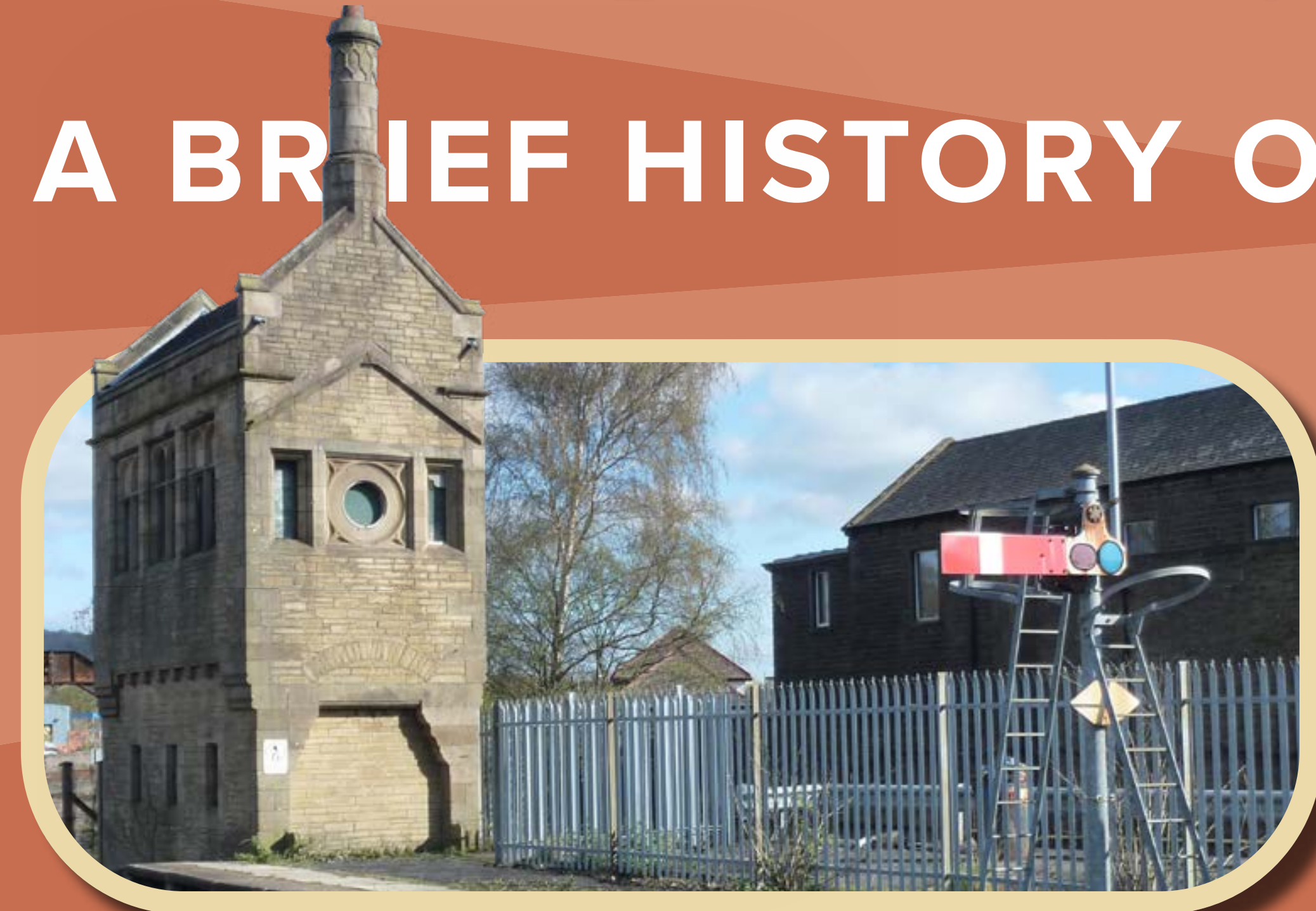
The grade II-listed Furness Railway signal box built in 1882 still stands proudly alongside the old Furness platforms at Carnforth in 2019. It is constructed of York stone it has two storeys and a slate roof. The tall round chimney sits on an octagonal base and carved on the north side of the building is the Cavendish coat of arms. Photo courtesy of Brian Haworth
