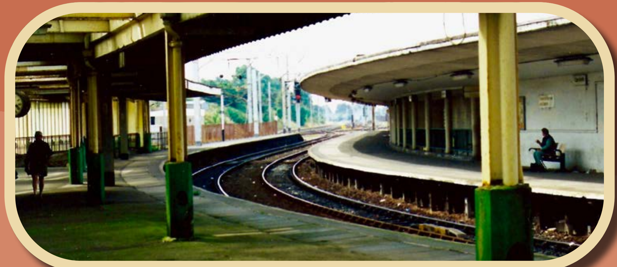
Carnforth station took on an air of neglect once the main-line platforms were removed. Its condition continued to deteriorate and by 1990 its buildings were at risk. The Furness platforms are captured in 1990. Photo from The Gerald Townson collection
